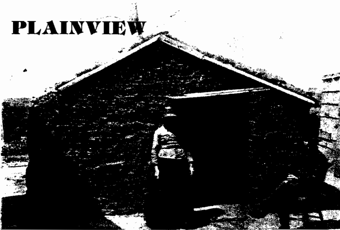
James Pendergast (born 1836, died 1904), built this sod house for his wife Margaret upon their arrival in Nebraska in the 1870s. It was located two miles east and one mile north of the Village of Plainview. [Ray Pendergast]
