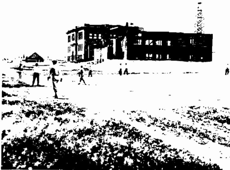
Below: Baseball players work out as the second new school building is being constructed, 1920.
